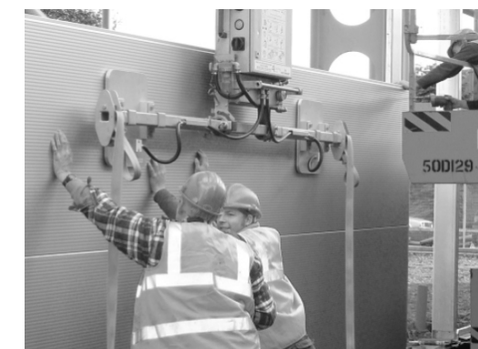
Fig. 2.5: Setting horizontal panels with vacuum.
