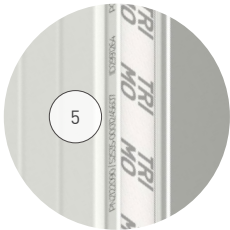
Fig. 3.8: Each panel is clearly marked with individual installation reference (example on the right). With Trimoterm FTV panels the reference is indicated on the internal side of longitudinal panel joint.
